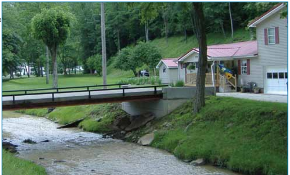
Figure 3.1-3. Bridge with wing walls direct water flow during high water to avoid washout of bridge approach and increase of water flow velocity. Guardrails on bridge safeguard traffic passage.
