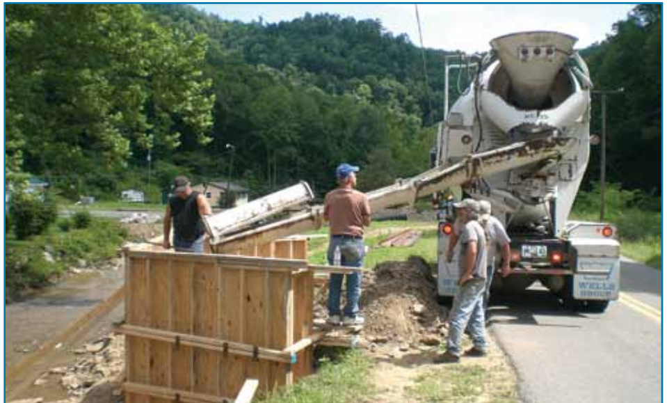
Figure 3.1-2. Concrete is being poured into a wood form for a cast in place reinforced concrete bridge abutment with wing walls. This abutment design was dictated by a short approach, but it is still high and set back far enough from the water channel to allow unobstructed water flow and safe passage to and from the property.
