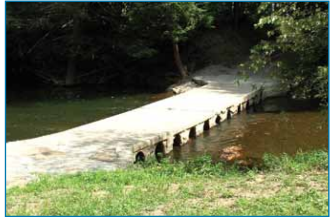
Figure 3.3-2. Concrete vented ford - this type of crossing has a low cost and low maintenance. Fish passage and scouring problems are a disadvantage as well as a danger to traffic during high flow periods.
